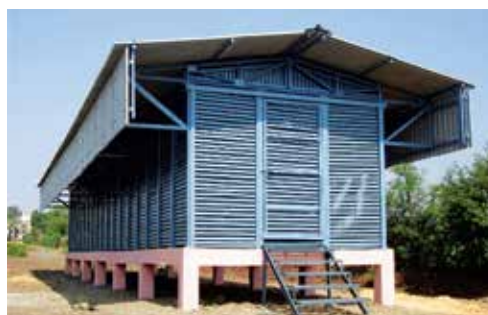
Bottom and side ventilated storage structure
